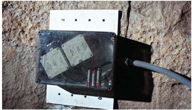
Figure 3 – Data logger, data-and-power-on-demand controller and AA batteries in enclosure on cave wall 6m above streamway
