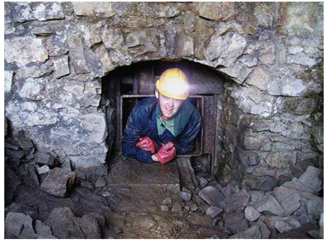
**Figure 7 – The OCAF gate with only fist-sized apertures between girders, which prevent bat flight**
