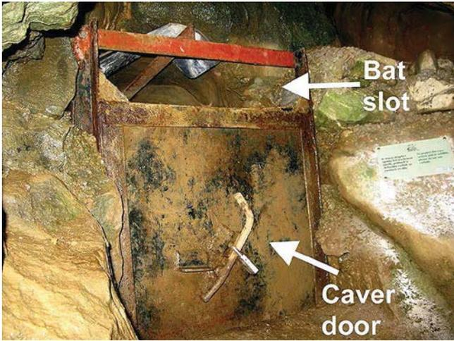
**Figure 6 – The 2002 Ogof Cnwc gate with wide slot for bat in-flight access**
